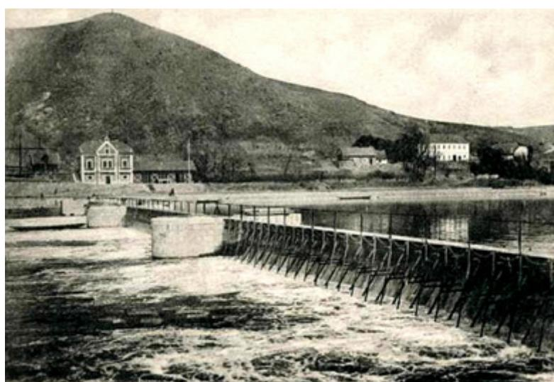
**Figure 4.** Needle weir in Klecany (1900).
